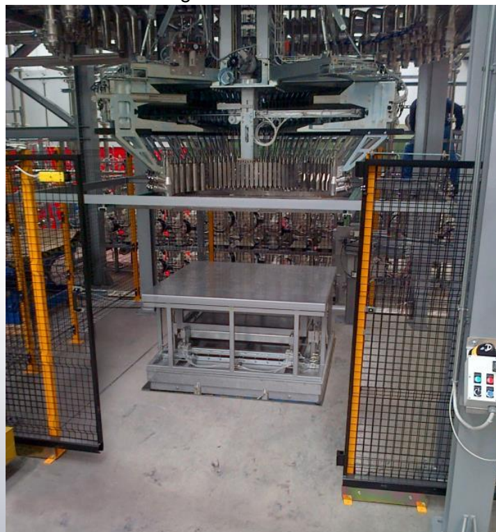
UWP above ground level
